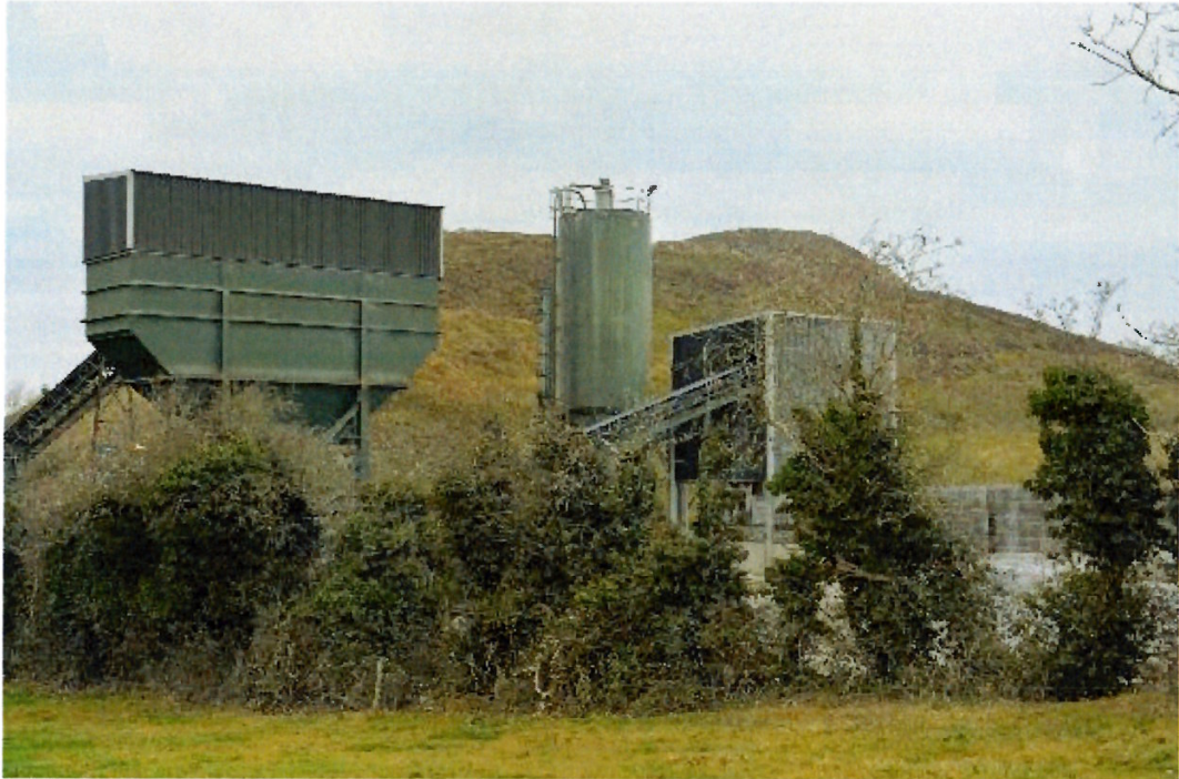
Concrete Batching Plant which was previously subject to a retention planning consent on the former Keegan site at Aghar a few miles away. This was moved to the Trammon site in May 2013. [ref.0395] ©
