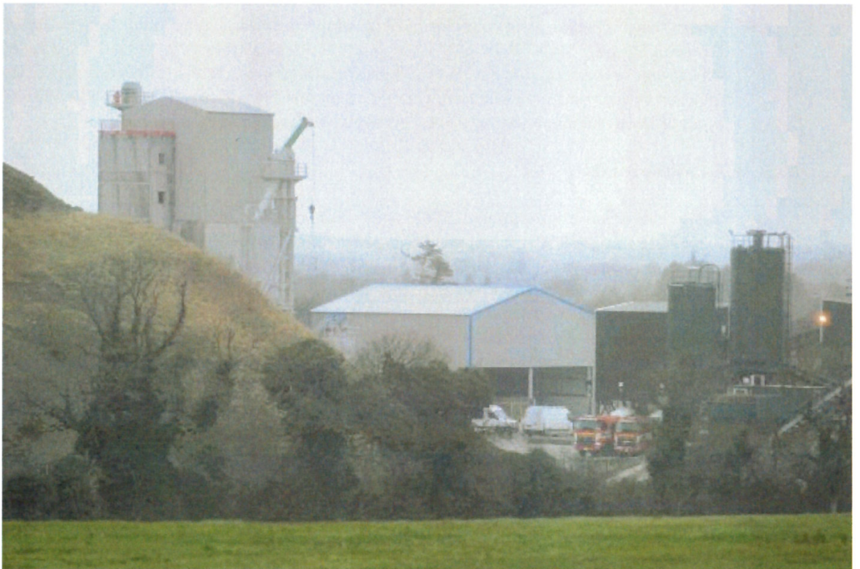
Construction of plant in 2016 without planning consent
